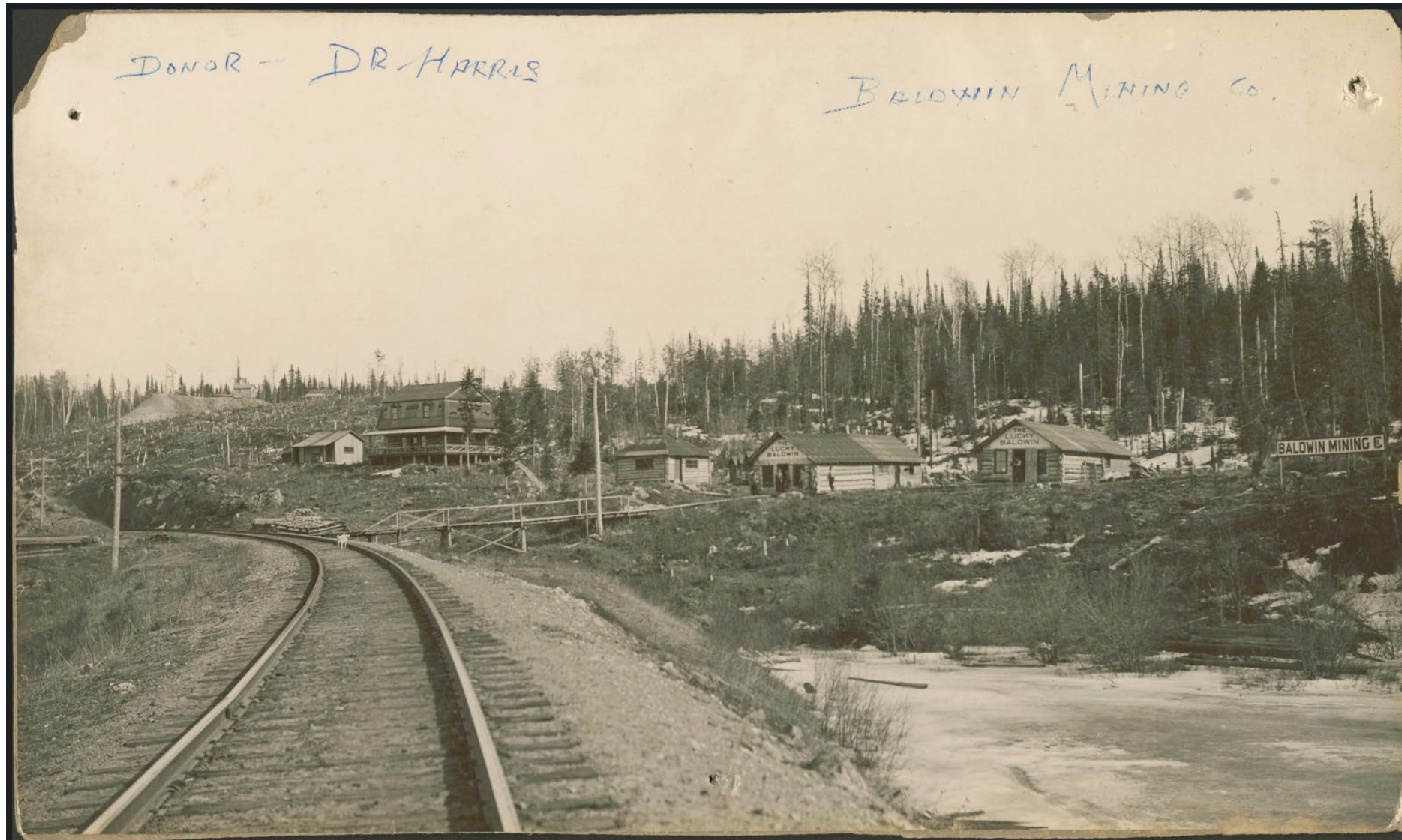
Figure 5: Historical photograph of the Baldwin mine-site office and associated buildings.
